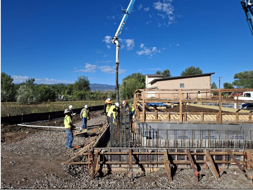
Foundation & Backwash Tank Concrete Placement
