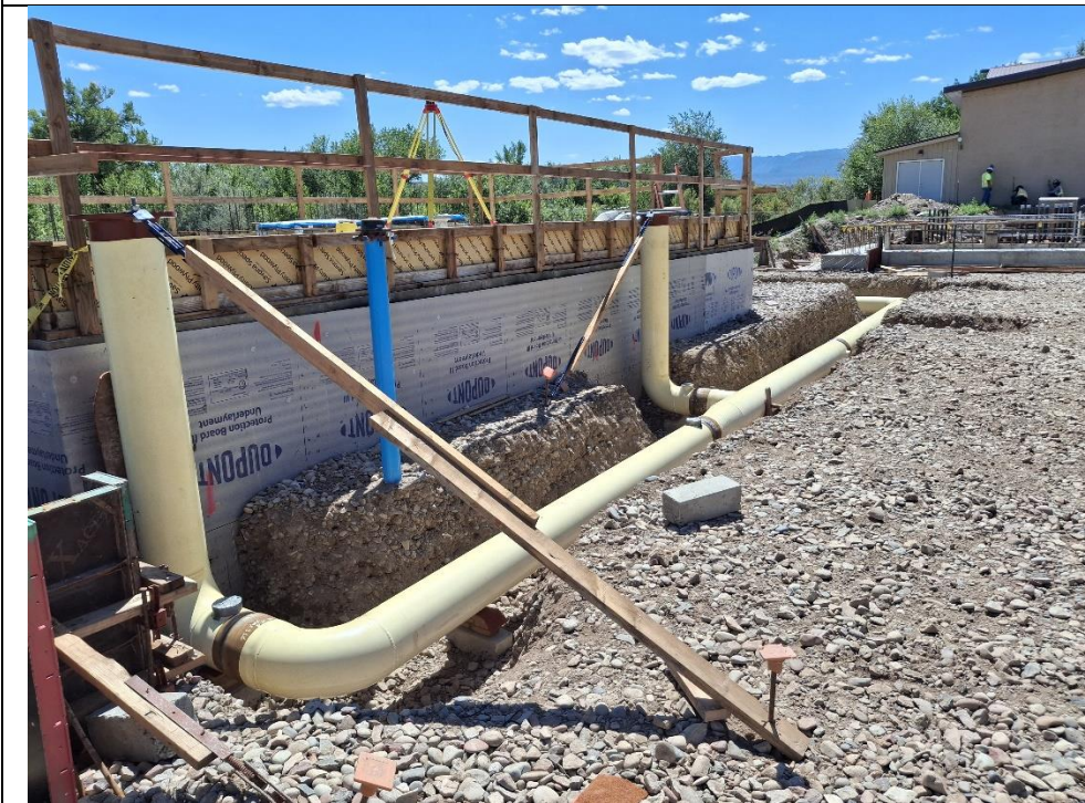
Underslab Process Pipe Install
