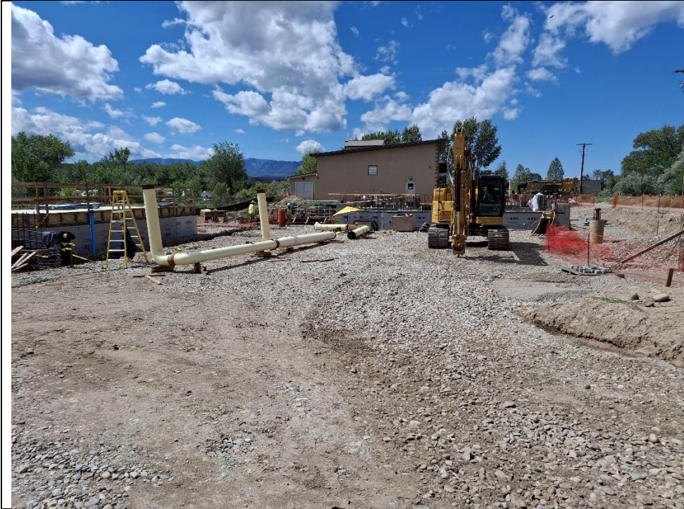
Underslab Process Pipe Welding & Install
