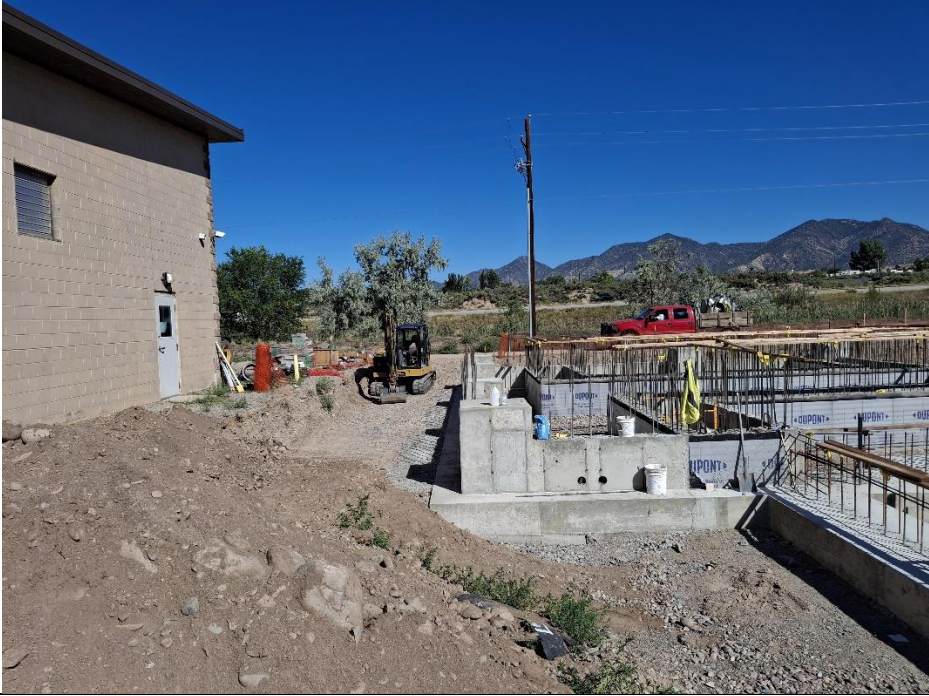
Yard Pipe Install
